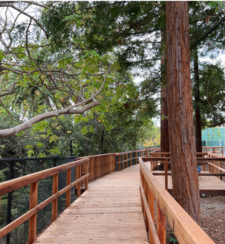
A deck constructed in an existing redwood grove at John Muir Elementary School transformed the forest into a flexible outdoor learning space.
