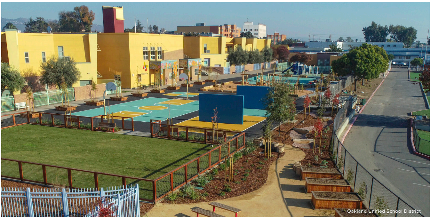
A bird's-eye view of OUSD's César E. Chávez Campus, a transformational project completed in 2021.
