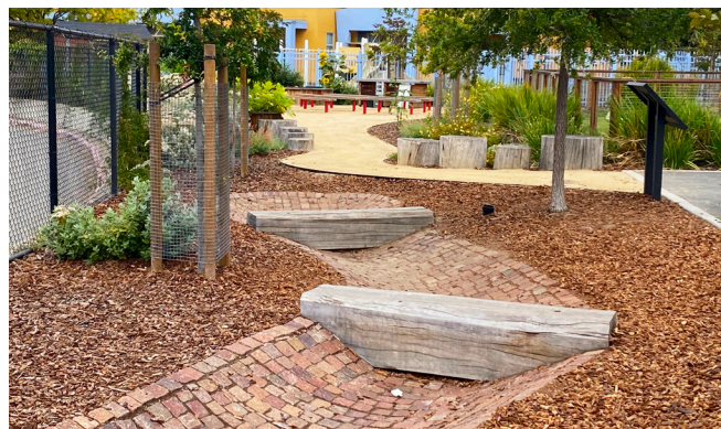
A rainwater catchment and infiltration swale surrounded by trees at OUSD's César E. Chávez Campus.
